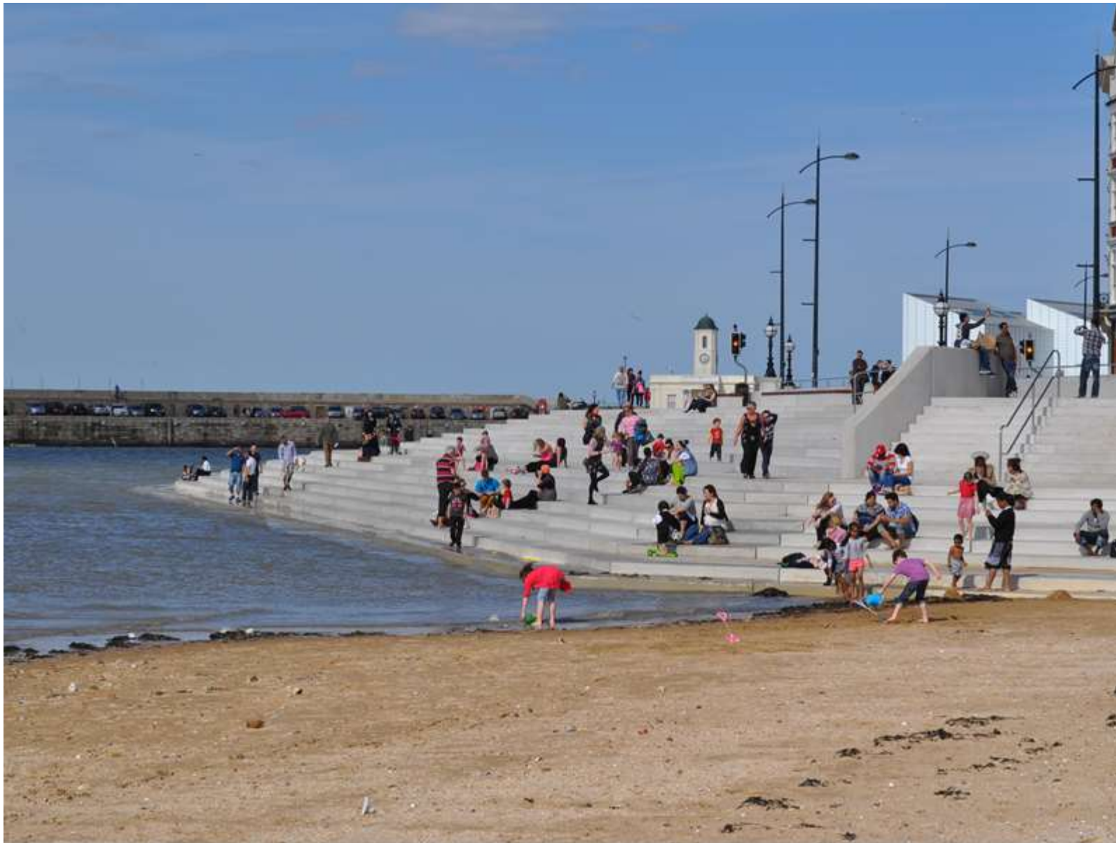
THE NEW KING'S STAIRS – MARGATE HARBOUR- re-linked Old Town with beach; popular meeting place WINNER OF CIVIC VOICE PUBLIC REALM NATIONAL DESIGN AWARD 2015
